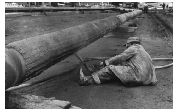
1963 - A workman applies a concrete coating to one of the pipes from Fawley to London to protect them from any damage which may occur on the river bed.
